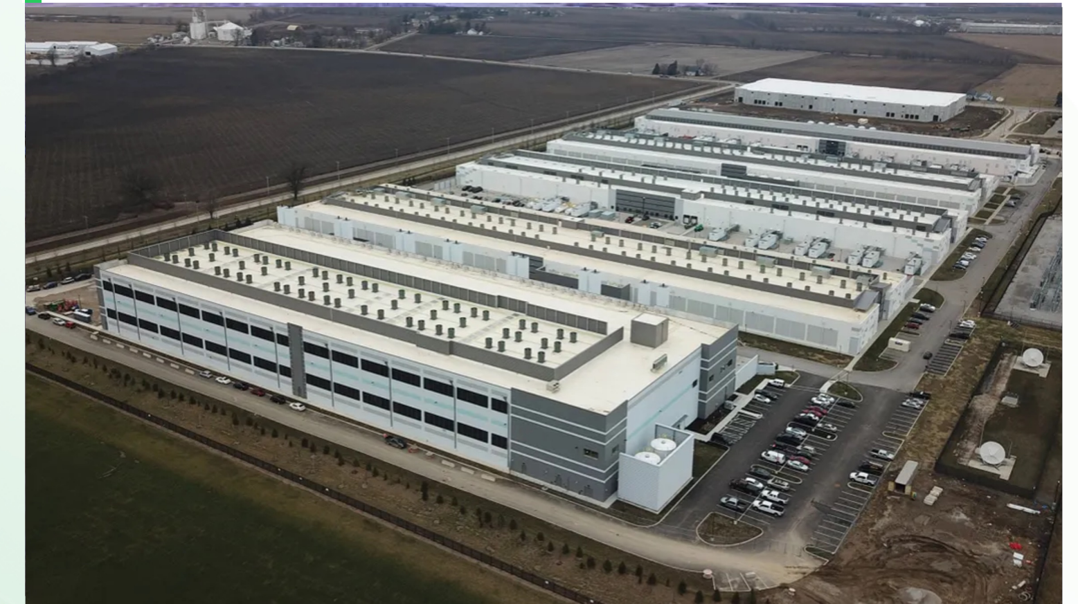
Baltimore Data Center
