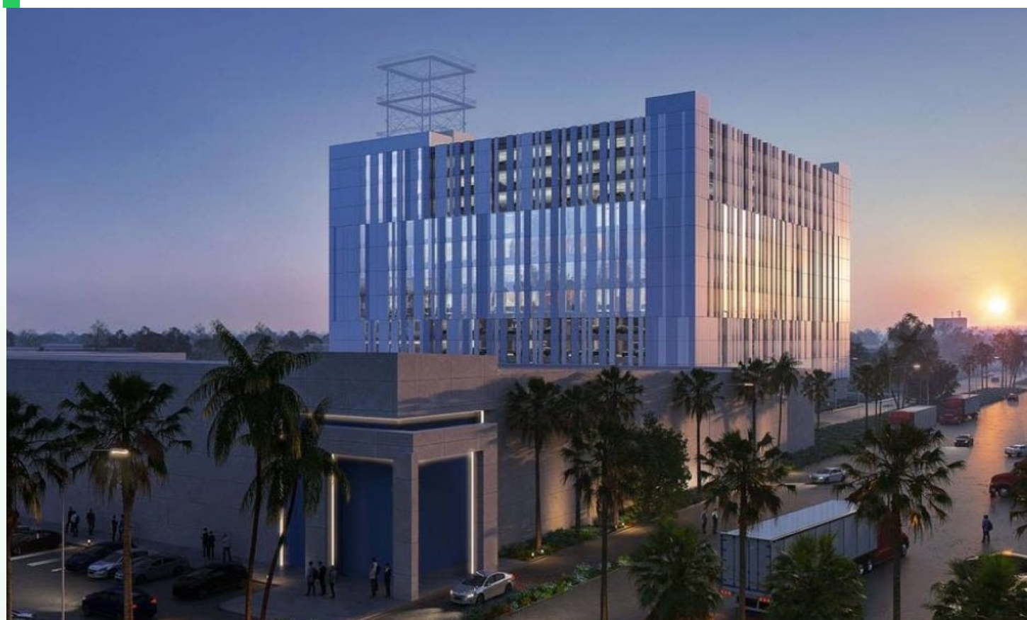
Miami Emergency Response Center
